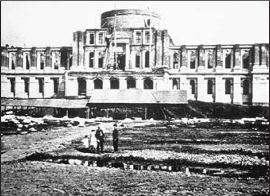
Capitol under construction in Sacramento, circa 1867
