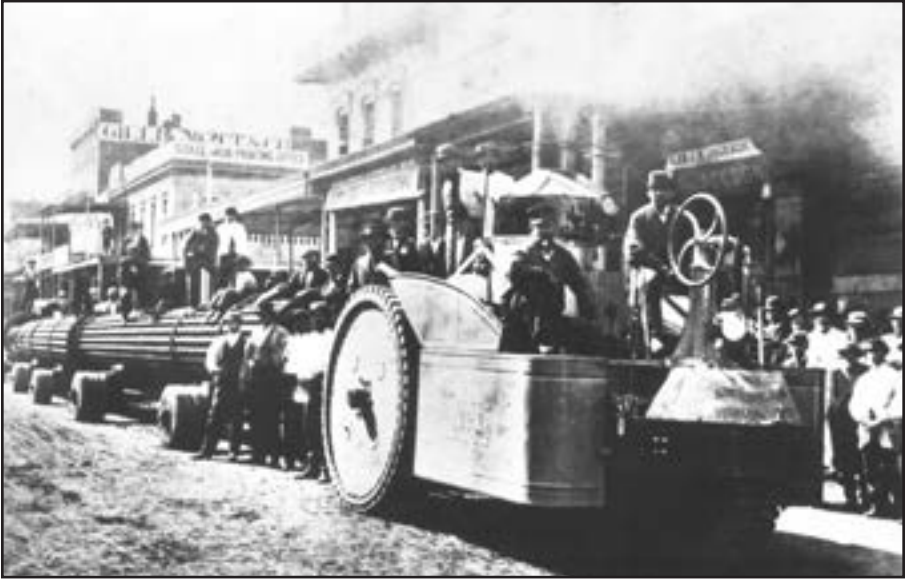
Steam-powered tractor pulls west entrance columns down J Street, circa 1870
