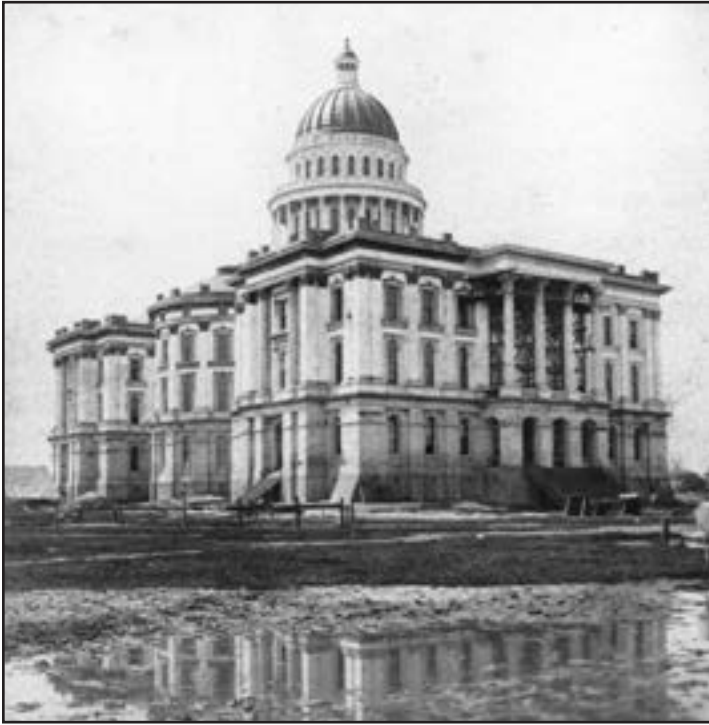
Capitol nearing completion, circa 1872
